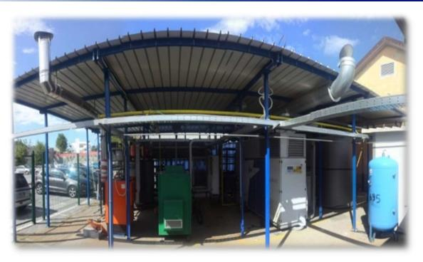
The validation phase will require the installation of cold thermal storage, fast-response HP (10 kWe), and compressor inlet heat exchangers arranged as in the picture to realize an Integrated Inlet Conditioning System.
